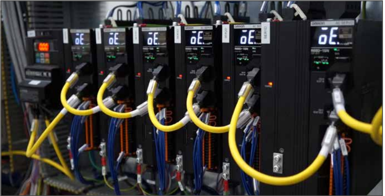
The OMRON NX701 controller manages 34 OMRON 1S servos and six 3G3MX2 inverters.
