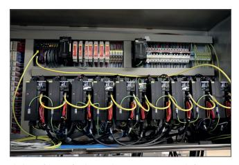
The basis of the retrofit solution is the Sysmac automation platform in addition to OMRON's 1S drives with continuous integration from the NX/NJ machine controller to the software.
