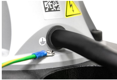
Figure 15: Securing the ground wire with the robot
